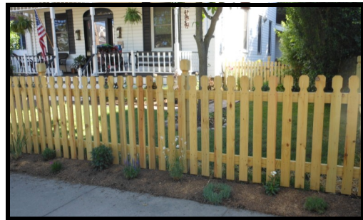
Picket Fence with Colonial Pickets and Post Tops
