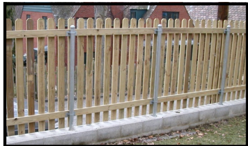
Wood Fence installed on wall with Steel Posts
